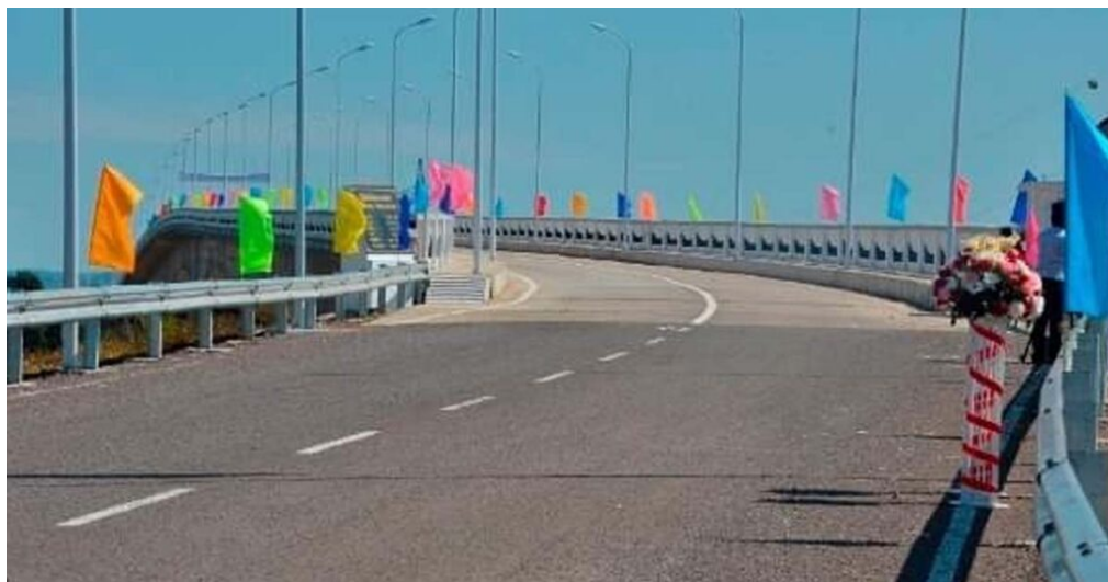
New concrete road opens in Don Khong.
